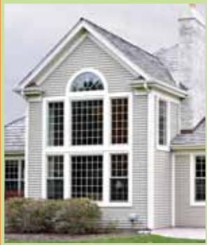
Windows Header, Sill and Jamb
