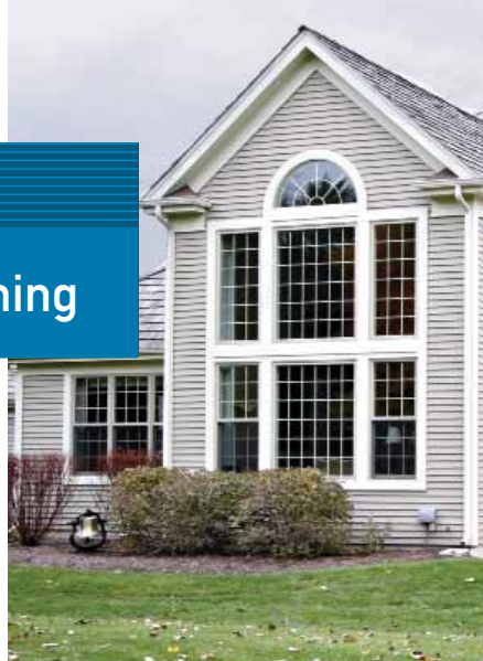
Windows Header, Sill and Jamb
